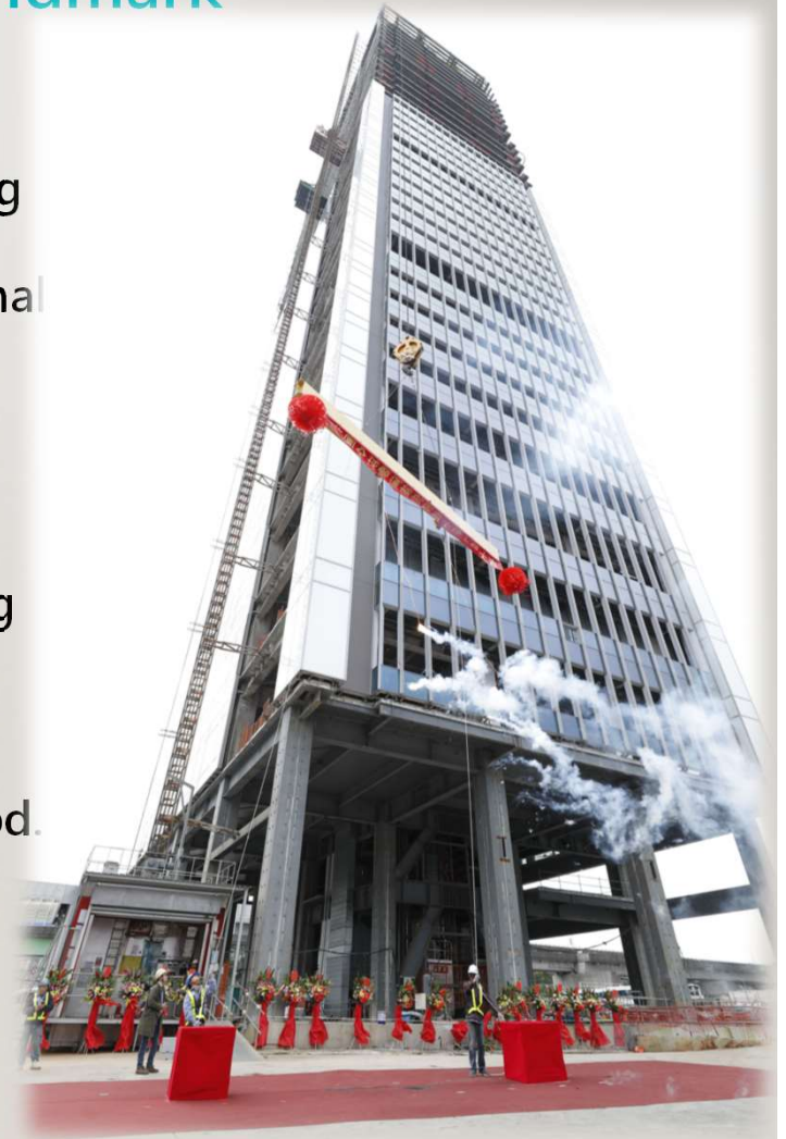
▲ Eastern Group Global Operations Headquarters Grace Building Topping Ceremony
